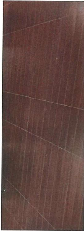
**INCORRECT INSTALL PATTERN:** Picture above shows the correct tile sizes, but installed in a grid instead of pattern specified in finish schedule
