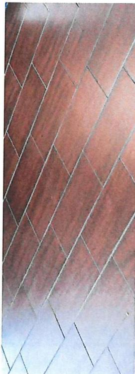
**INCORRECT INSTALL PATTERN:** Picture above shows only a single size of tile, not the mix of sizes specified in finish schedule
