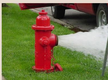
The Public Works Department Utilities Division will begin its annual hydrant flushing program in late March. This process moves water through the pipelines at a fast rate to clean the lines, clear stagnant water, and identify broken hydrants. Each hydrant is left open for approximately 2 to 3 minutes until the water runs clear. Crews will work in sections and the whole program takes about 3 weeks to
