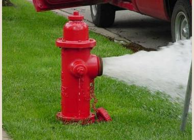
annual hydrant flushing program in late March. This process moves water through the pipelines at a fast rate to clean the lines, clear stagnant water, and identify broken hydrants. Each hydrant is left open for approximately 2 to 3 minutes until the water runs clear. Crews will work in sections and the whole program takes about 3 weeks to complete, depending on weather.
