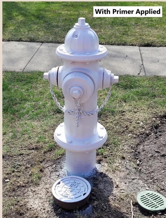
Fire hydrant painting began last week. Contracted crews are removing layers of paint down to bare metal, priming, and painting selected fire hydrants. The area targeted for this year is roughly from Dundee and Rand Roads south to Northwest Highway and Lincoln Street between Smith Street and Rohlwing Road.
