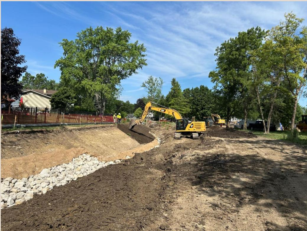
Work continues on the Salt Creek Streambank Stabilization project. Grading and armor stone installation along the south bank are underway. Work on the south bank east of Clark Drive will continue for the next week, depending on weather.
