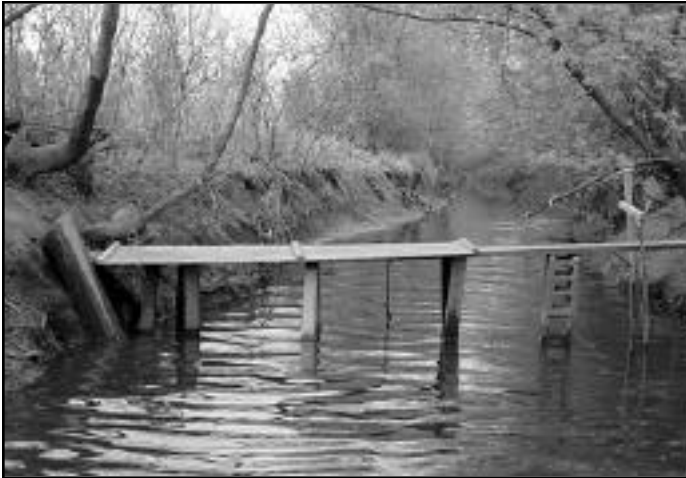
Whoever built this bridge no doubt had lots of fun doing it, but when the water level rises the bridge will become floating debris that will cause flooding downstream.
