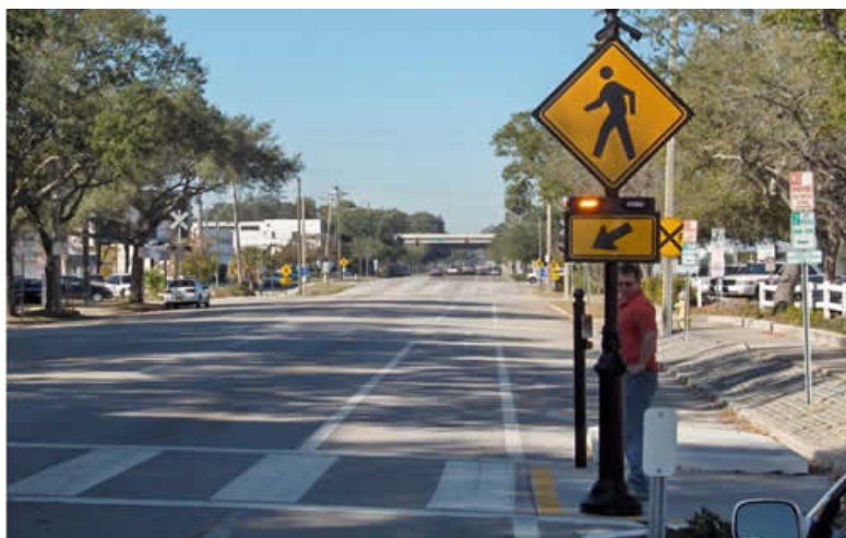
Figure 2.13. Rectangular Rapid Flashing Beacon. Courtesy FHWA.
