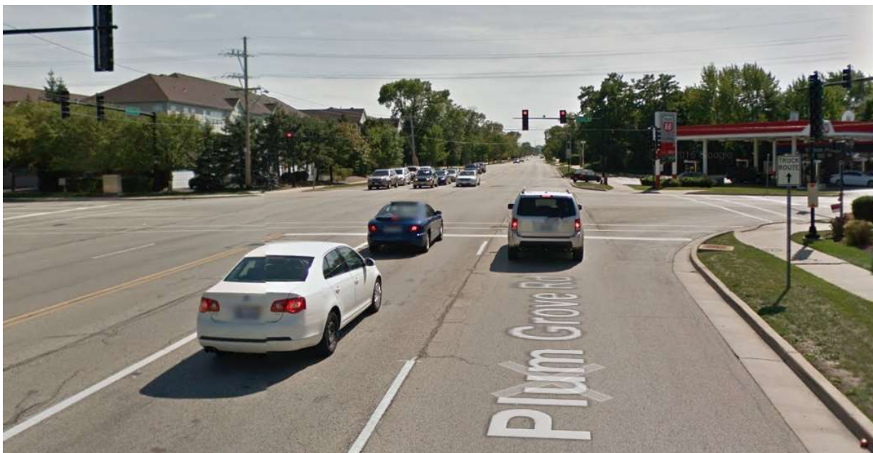
Illinois Avenue at Plum Grove Road, Eastbound Approach
