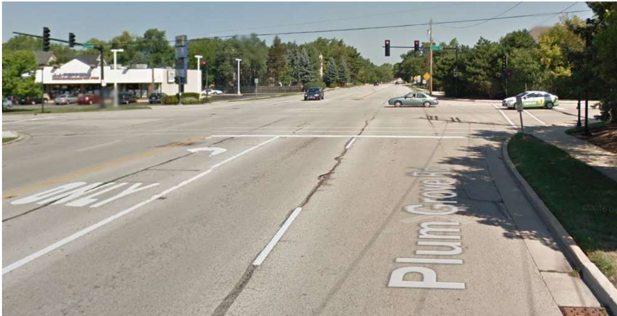
Illinois Avenue at Plum Grove Road, Southbound Approach
