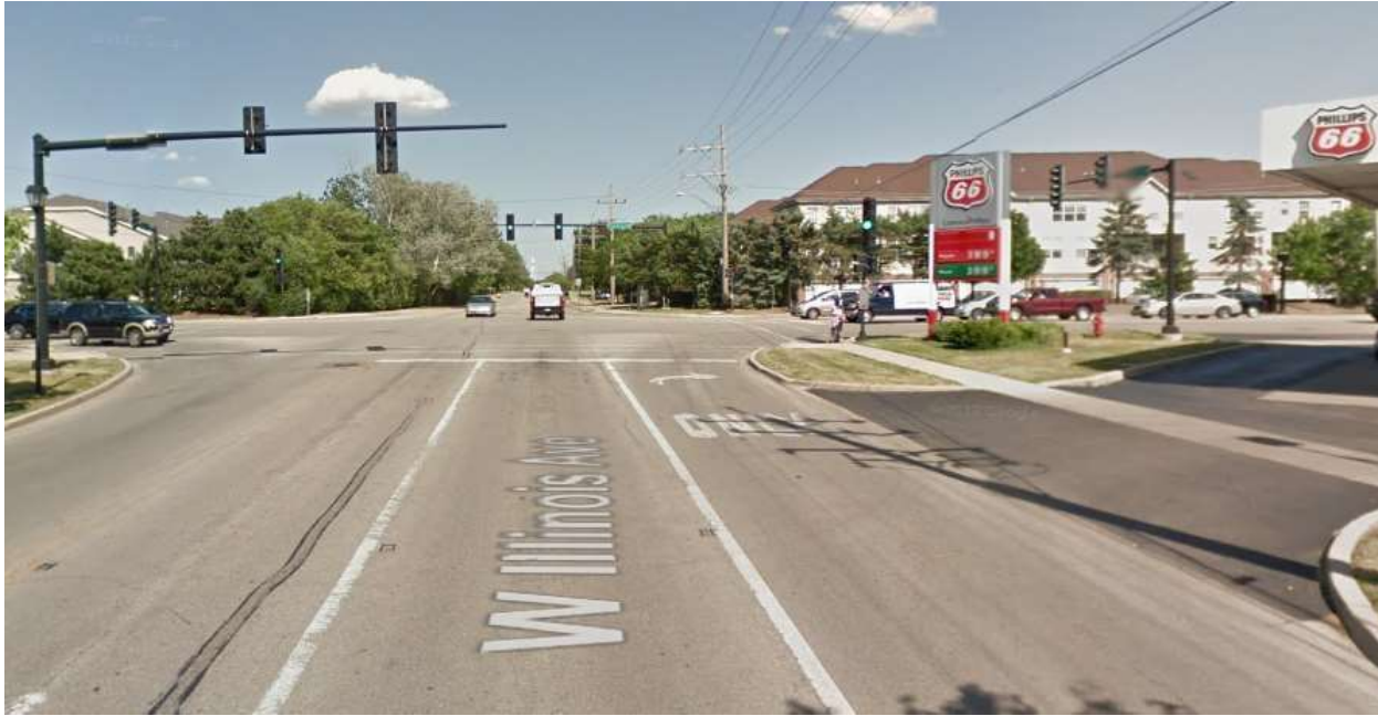
Illinois Avenue at Plum Grove Road, Westbound Approach
