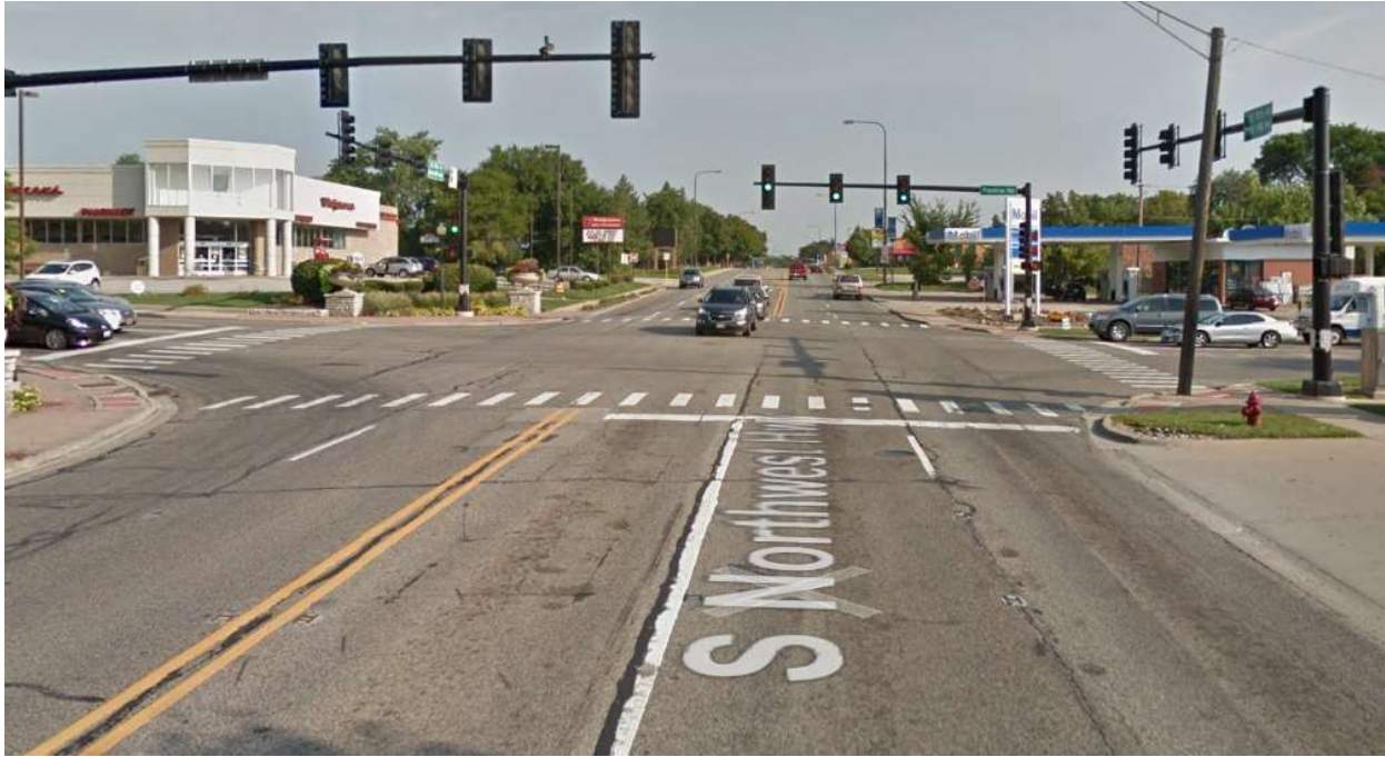
US Rte. 14 (Northwest Hwy) at Palatine Road, Southbound Approach
