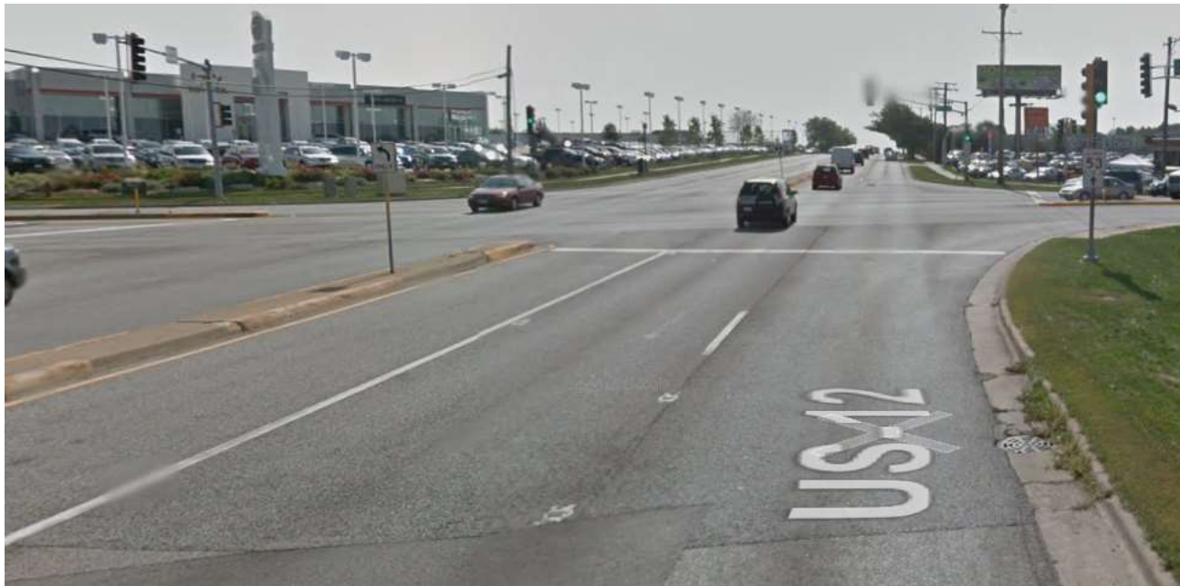
US Rte. 12 (Rand) at Hicks Road, Northeast bound Approach
